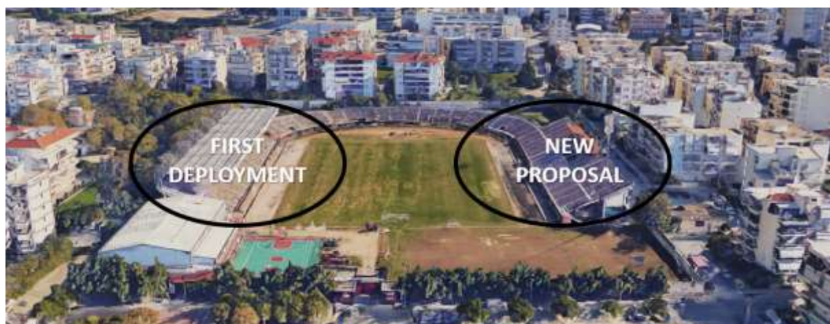
Figure 1. General view of the stadium: IoT deployment enlargement
